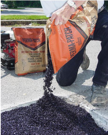
Clean out only large, loose aggregate from pothole. Place Perma-Patch in hole and compact by driving over the patch with a truck, hand tamper or use a vibratory plate compactor. For deep potholes, place Perma-Patch in 3" lifts and compact each lift.
