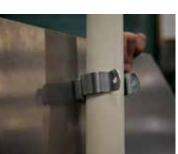
Step 4: Tighten with screws supplied
