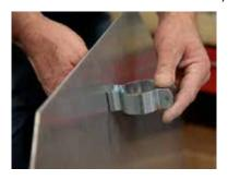
Step 3: Widen the opening of the bracket and make sure it wraps around the post
